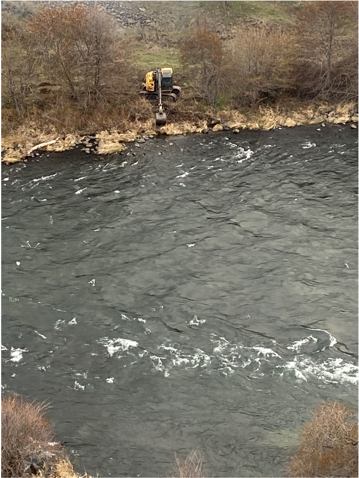
Figure 4 Feb 2022 Excavator Pulling Vegetation/Trees from River
