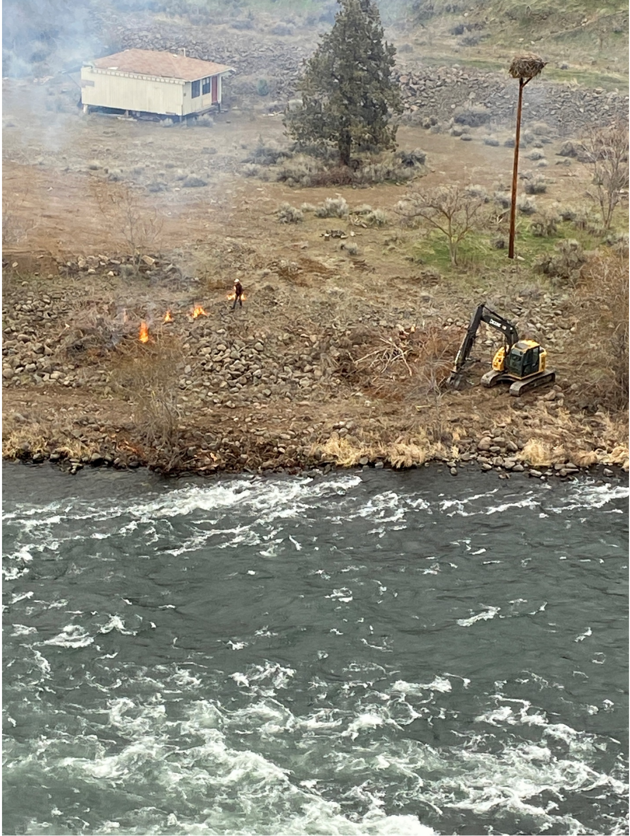
Figure 3 Feb 2022 Excavator Pulling Vegetation/Trees from River and Burning Vegetation
