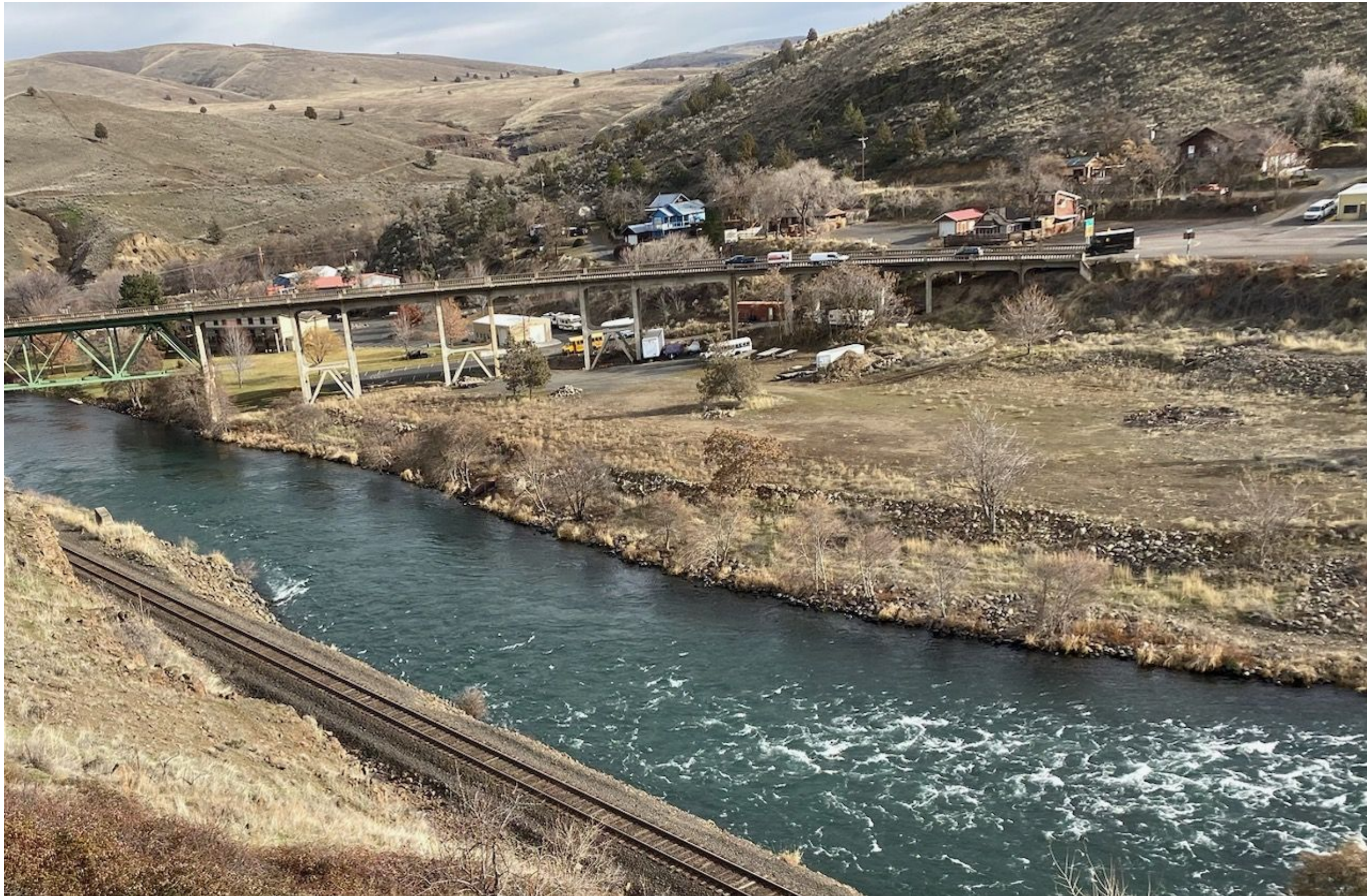
Figure 7 Feb 2023 After Removal of Vegetation/Trees From River – 1 year later
