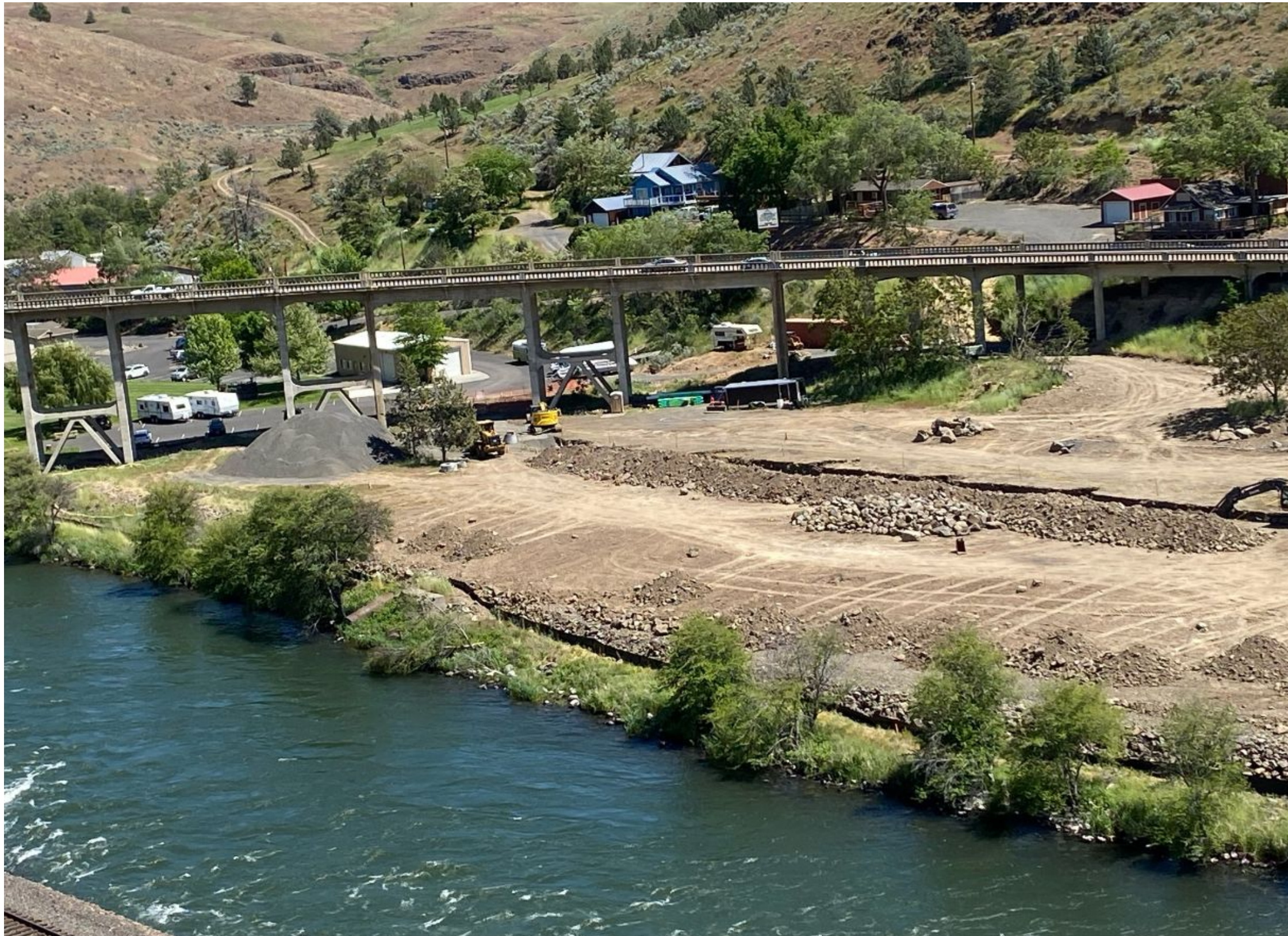
Figure 12 May 2024 During Construction
