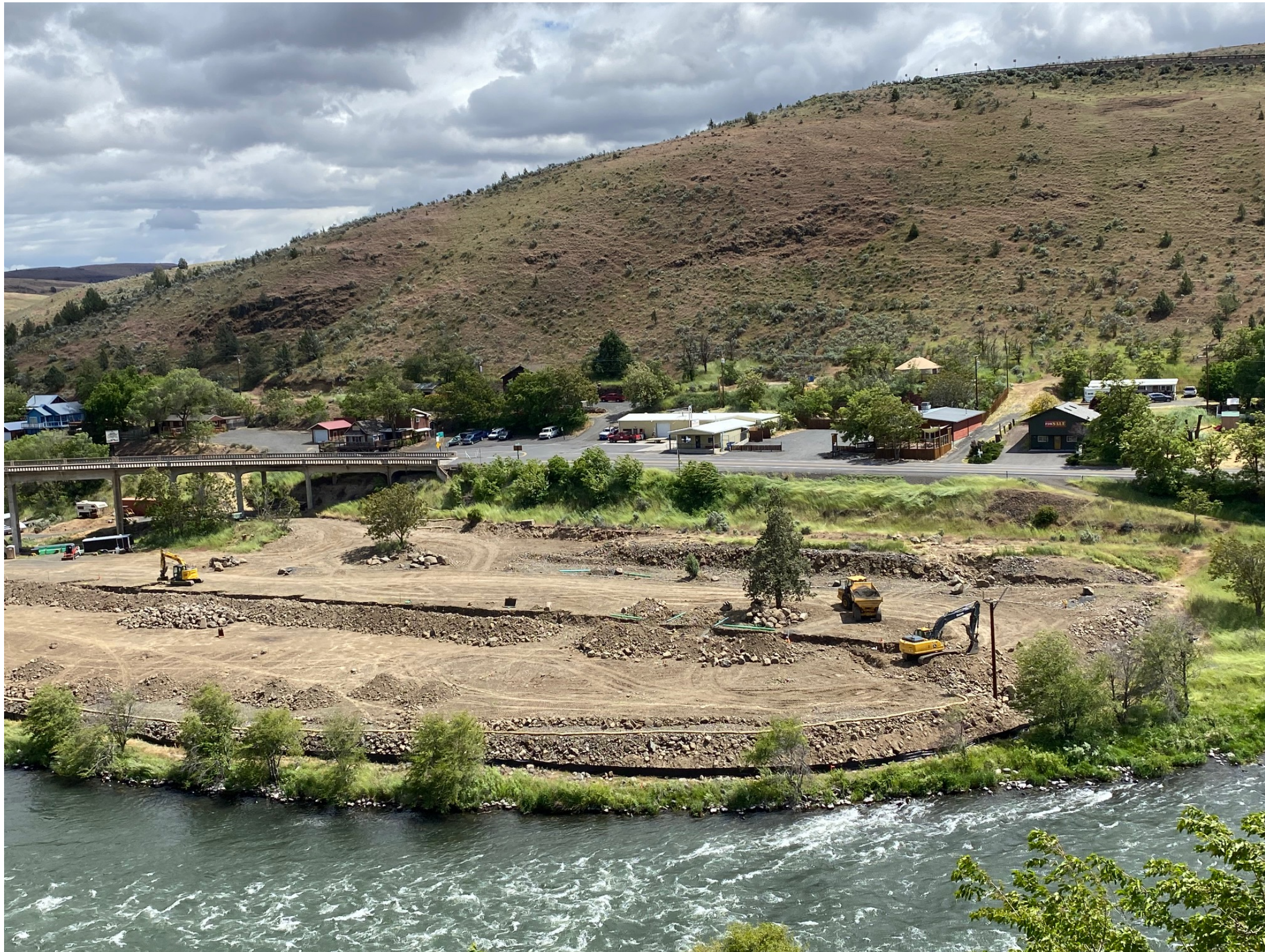
Figure 10 May 22 2024 – Old Osprey nest removed – new one installed at property marker
